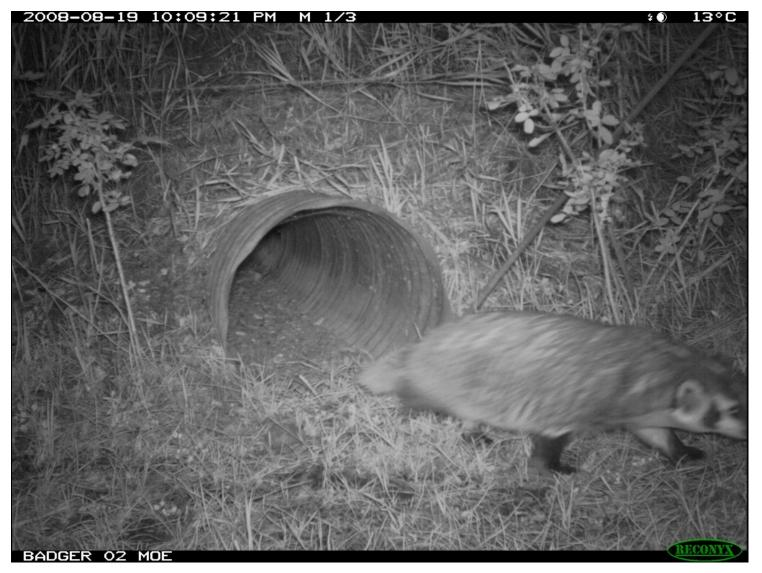
Figure 3.2. Suitable existing underpass structure (500 mm corrugated pipe) with earth substrate bottom used by badgers to pass under Highway 97 north of 100 Mile House BC, Canada, 19 August 2008.
